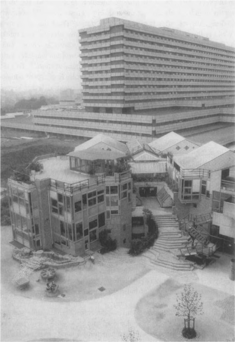
Figure 4.2. Catholic University of Louvain, Brussels, Belgium, Atelier Lucien Kroll. Symbolizing what the medical students were trying to overcome in conceiving new forms of medical practice, the rigid and banal style of the hospital (background) stands in stark contrast to the creative interplay of form, color, texture, and material of Kroll's contribution. (Photo by Thomas A. Dutton.)
