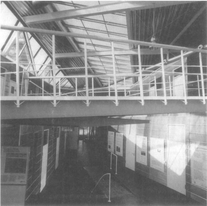
Figure 6.2. Interior, Hysolar Institute, University of Stuttgart, Germany, Behnisch and Partners. (Photo by Christian Kandzia. Used by permission.)
